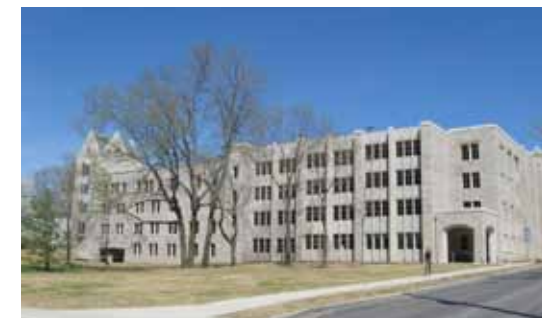
Atwater Parking Garage
