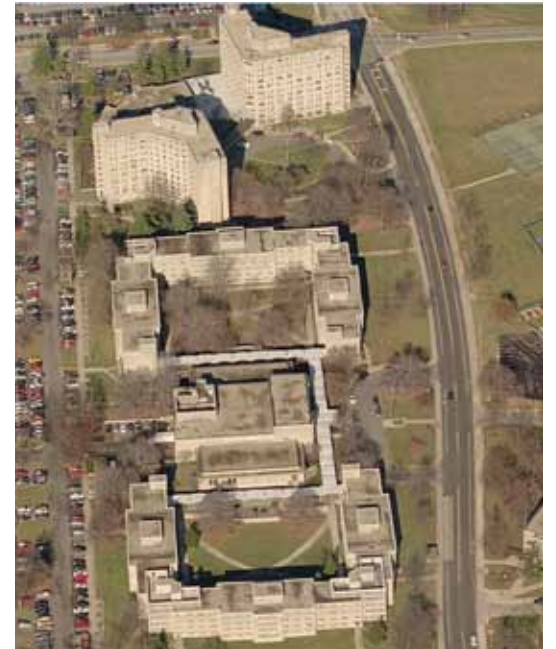
Aerial View of Briscoe and McNutt Dormitories
